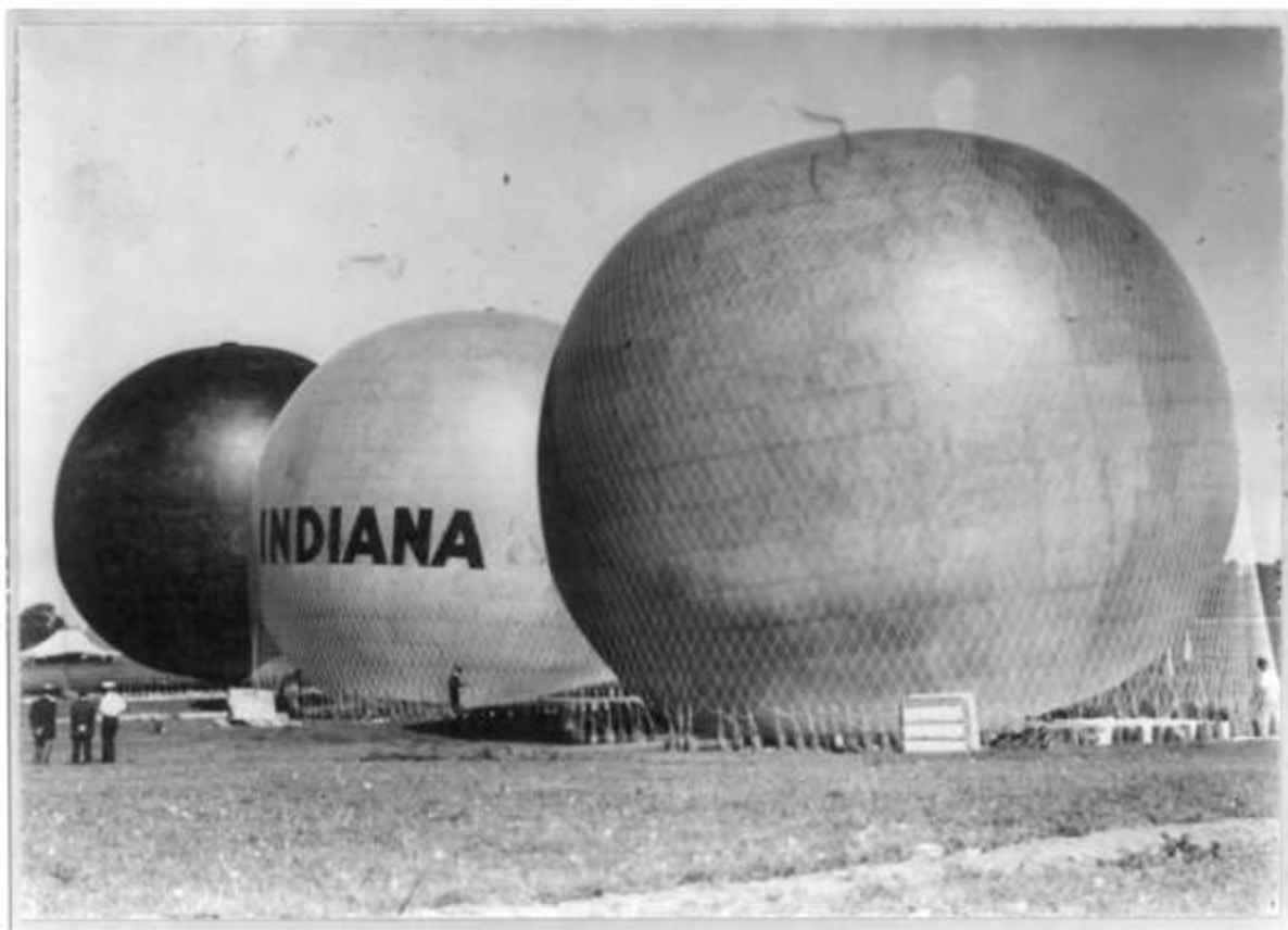
Balloons: Chicago, Indiana, and Hoosier netted down to ground prior to the National Balloon Race in 1909 starting at the Indianapolis Motor Speedway.
