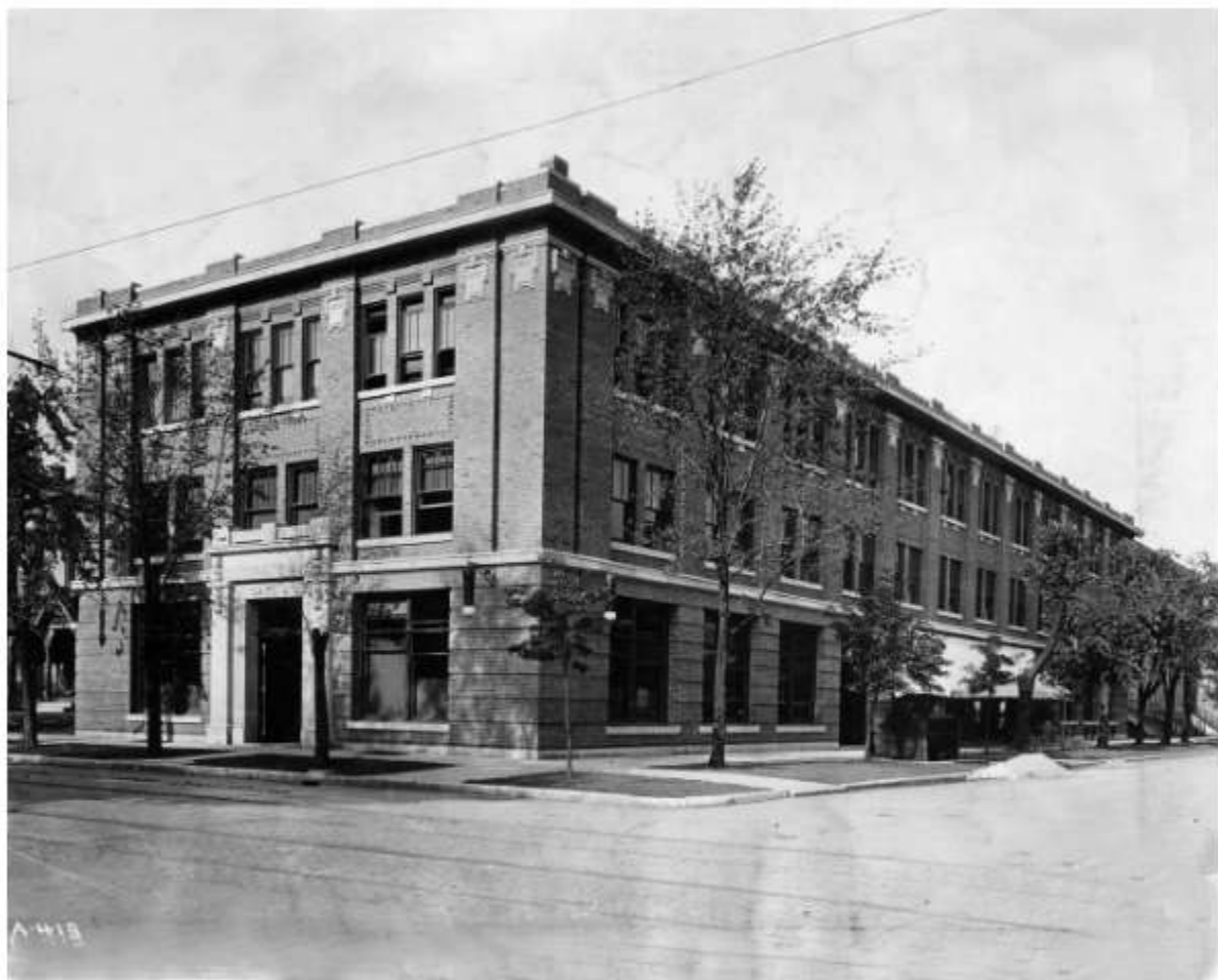
This view of the Star building, 301 North Pennsylvania Street, was taken shortly after it was built in 1907.
